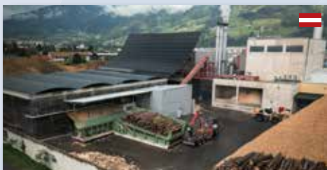
Biomass heating plant - Austria
