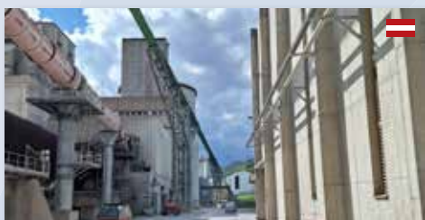
Cement plant - Austria
