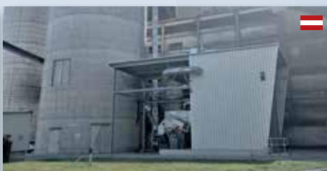
Cement plant - Austria
