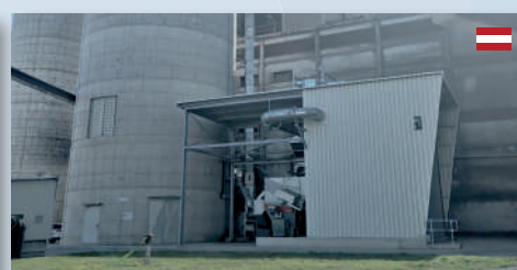
Cement plant - Austria
