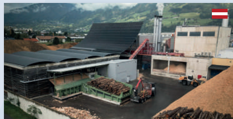
Biomass heating plant - Austria
