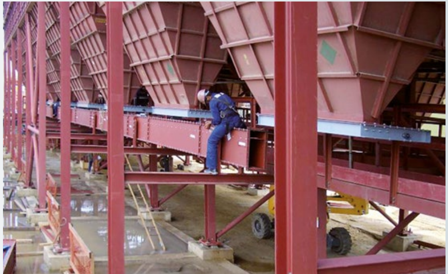
Installation of a chain conveyor in a filtration system
