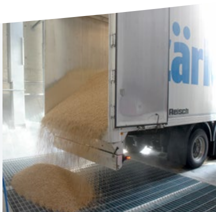
Intake pits for lorry and train unloading
