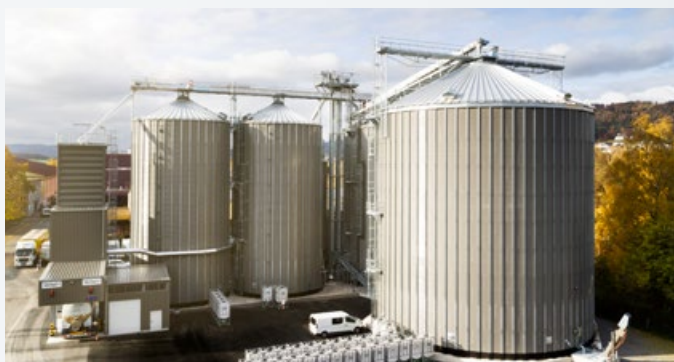
9000 t pellet storage with one receipt and two loading terminals
